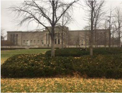
Figure 1. The Original Nelson-Atkins Building, 1933.
